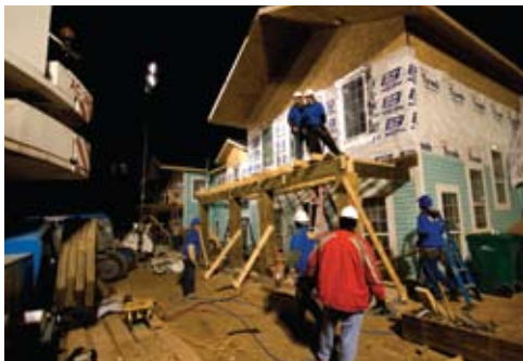
Top: Day three of the build: SIP wall panels go up and flooring goes in on the second floor.
